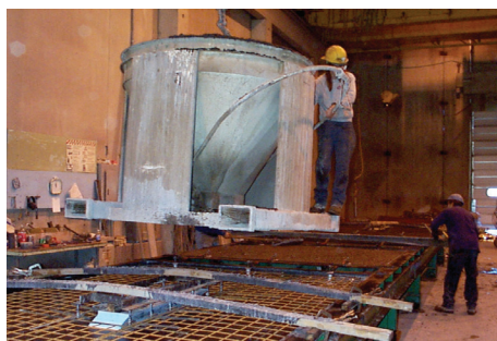
Figure 7.9 – Negative Cast Method. Concrete is poured and vibrated over the panels. A slurry bond coat consisting of LATICRETE® use 3701 mortar bed.
