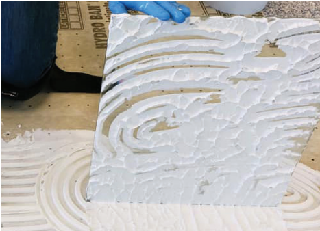
Figure 9.8 — Insufficient adhesive mortar coverage. Removal of a tile reveals many voids that are present in the hardened thin set mortar. Trowel ribbons are inconsistent which will also lead to poor coverage and mortar transfer to the backs of the large format tile/stone.
