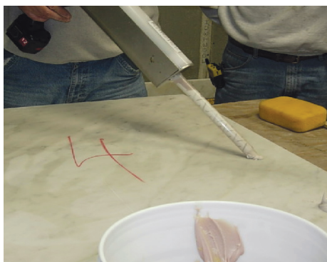
Figure 9.17 — Epoxy spot bond (e.g. LATAPOXY® 310 Stone Adhesive) adhesive is applied to the back of the stones with an automated epoxy mixer / applicator. A minimum of 10% adhesive coverage is generally required. The LATAPOXY 310 Stone Adhesive is available in standard grade (maximum working time of 45 minutes) or rapid grade (maximum working time of approximately 5 minutes).
