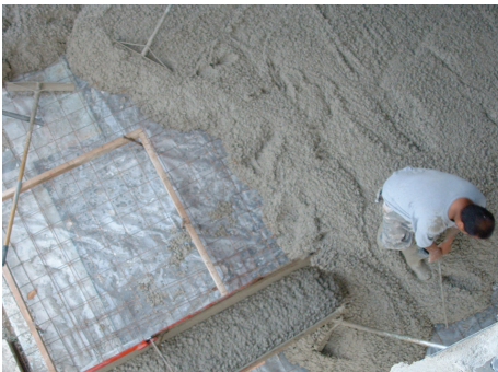
Figure 4.16 — Placement of vapor barrier/vapor retarder over blotter layer/directly under the concrete pour. Notice the mechanic pulling the reinforcement wire to the middle of the concrete pour.
