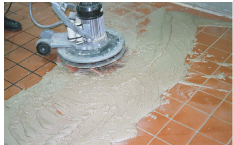
Figure 10.26 – Grout Spreading Process.
