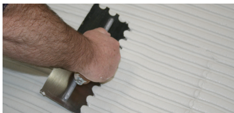
Figure 9.5 — Trowel applied medium bed mortar with a 3/4" (19 mm) loop notch trowel used for large format tiles or stones. Trowel medium bed mortar in one direction holding trowel at a 45 degree angle. Notice the full ribbons of mortar that are left behind.
