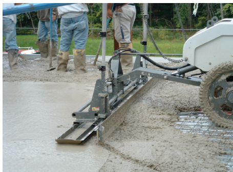
Figure 4.12 – Placement and screeding of concrete slab over steel pan.
