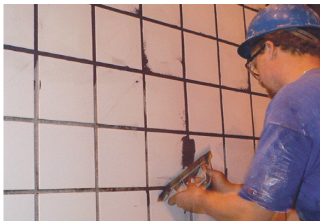
Figure 7.10 — Once the tiled panels are cured, the grouting process can begin. These panels are grouted with SPECTRALOCK® PRO Grout*.
