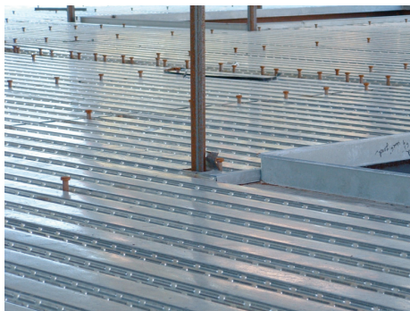
Figure 4.28 — Steel Pan Showing Placement of Shear Connections and Edge Detail.
