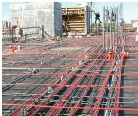
Fig. 4.24 — Post Tensioned Concrete Slab — Notice the Orange Tensioning Cables That Will Run Throughout the Concrete Slab — Photo Courtesy of SunCoast Post Tensioning Company.
