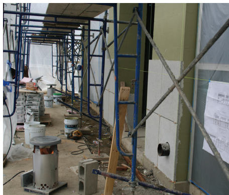
Figure 10.1 — Exterior façade work in temporarily heated, tented area in the middle of winter.
