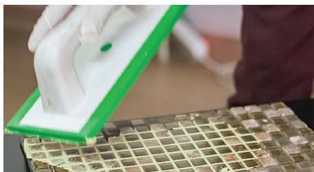
Figure 9.23 — Spreading of epoxy grout.
