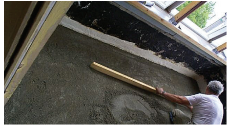
Figure 4.10 — Installation of an unbonded wire reinforced mortar bed.
