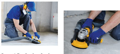
Figure 4.7 — Dustless Grinding.
