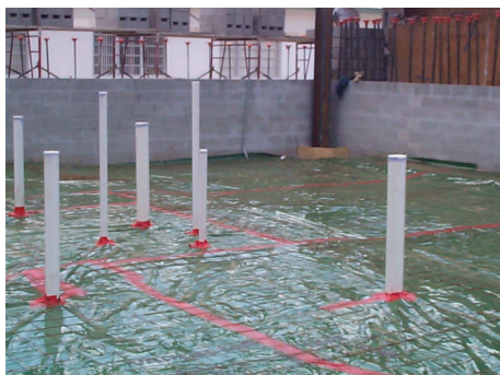
Figure 4.14 — Proper vapor barrier/vapor retarder placement.
