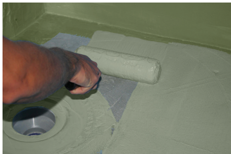
Figure 8.2 — Liquid applied membrane applied to concrete substrate.
