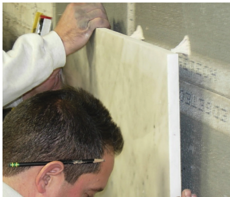
Figure 9.18 — Stones are then placed, leveled and plumbed to the required finish.
