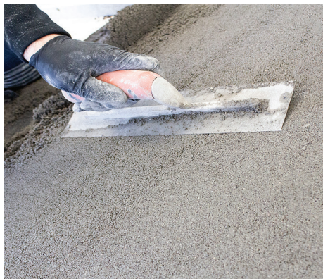
Figure 9.13 — Tile mechanic screeding a mortar bed.
