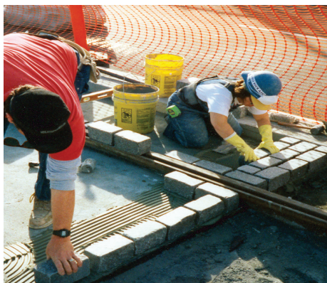
Figure 9.12 — Fisherman's Wharf Railway Paving Project, San Francisco, CA. Granite pavers installed over cured bonded thick bed mortar with LATICRETE 211 Powder mixed with LATICRETE 4237 Latex Additive. Pavers are placed between the rail tracks.
