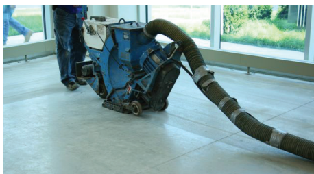
Figure 4.8 — Shot Blasting Machinery Creates a Concrete Surface Profile to Improve Adhesion and Remove Contaminants.
