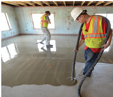
Figure 9.19 — Application of self leveling underlayment over a primed concrete substrate.
