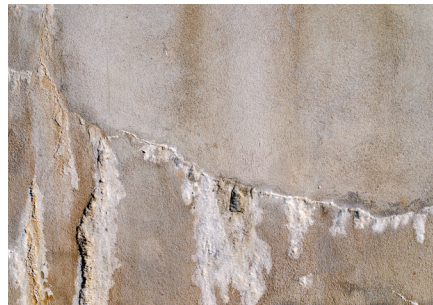
Figure 4.23 — Presence of Efflorescence on surface of concrete slab. Moisture migration through the slab can carry destructive salts to the surface of the concrete slab.
