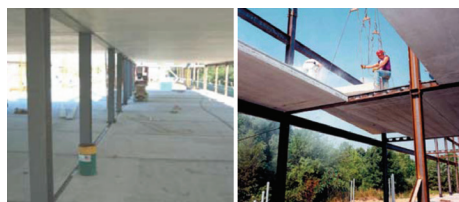
Figure 4.27 — Pre Cast Concrete Planks. Planks rest and are supported by a flange attached to the steel girders. The planks are hoisted into place by a crane and mortared to the beams and to each other. Photo courtesy of Girder Slab Technologies LLC.
