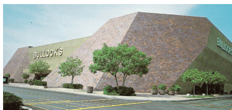
Figure 9.1 — High adhesive shear and tensile strength to resist seismic movement. Before photograph of the Bullock's building prior to the Northridge, CA earthquake in 1994. Tiles were installed on the exterior façade with LATICRETE® 4237 Latex Additive mixed with LATICRETE 211 Powder over LATICRETE 9235 Waterproofing Membrane.
