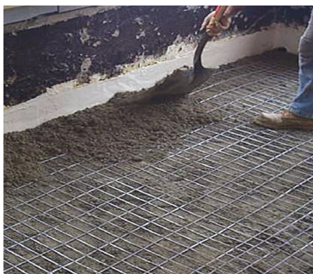
Figure 9.11 — Example of a non-bonded, wire reinforced mortar bed. Wire mesh is placed in the middle of the mortar bed and lapped together to ensure continuity. Notice that the mortar below the wire mesh has been compacted, thus ensuring that the entire mortar bed is compacted properly.
