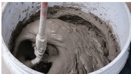
Figure 9.3 — Mixing of liquid latex fortified portland cement medium bed mortar.
