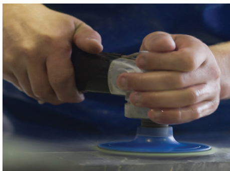
Figure 9.16 — Stone is prepared for installation by the epoxy spot bond method. Stone back is roughened at the adhesive connection points then washed and allowed to dry.
