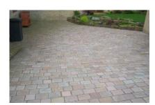
For the optimal results, paver joints should be a minimum of 1/4" wide and at least 1"
